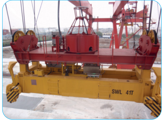
spreader power cables
